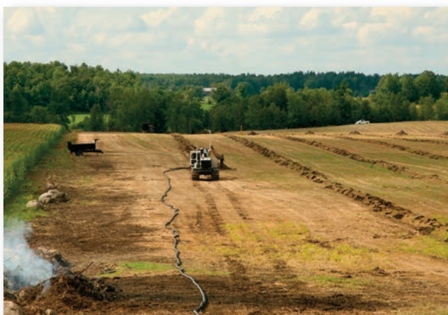
Drainage tiles, such as those being laid above, allow water to drain more quickly from fields into nearby waterways. They can also carry manure that percolates down with the water into the tiles. Photo: Zigzag Mountain Art/Shutterstock
